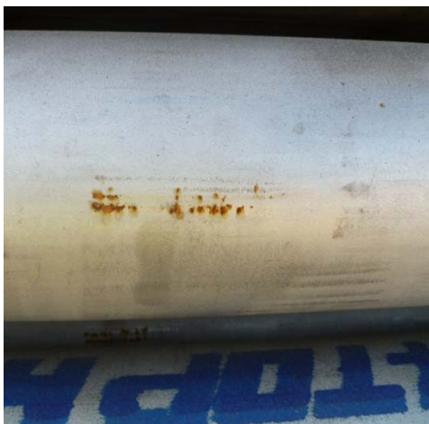
Pic # 1 Superficial contamination
